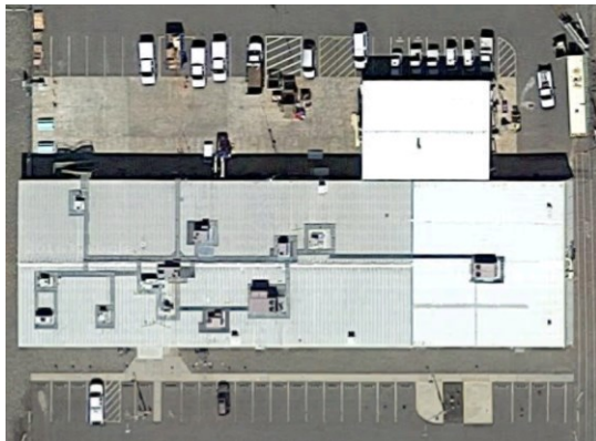
Figure 10. External view of the building on PNNL campus
